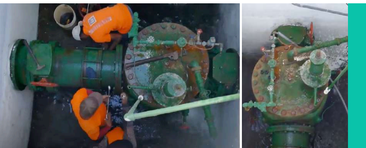
The old valve is being removed
