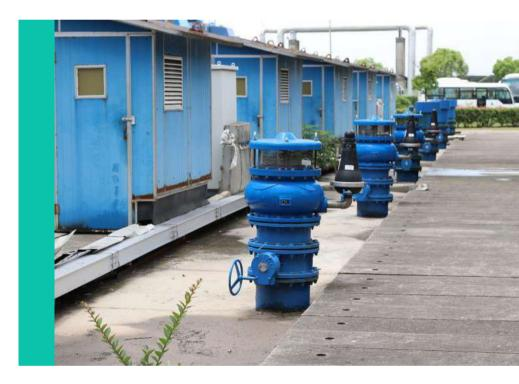
Following an energy analysis using ARIavCAD, A.R.I. supplied five units of 16" VB-060 vacuum breakers, and a D-025L combination air valve in a specially-designed sea water specification. This solution successfully discharges the huge volume of air entering the system via the pumps and prevents vacuum build up, while an advanced rolling sealing mechanism prevents orifice blockage, venting large air capacities during operation, all while withstanding the harsh water conditions.
